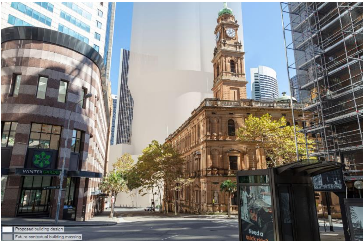
Figure 22 – View south-east from Bent Street toward the subject site showing indicative massing of the proposed building in context.
