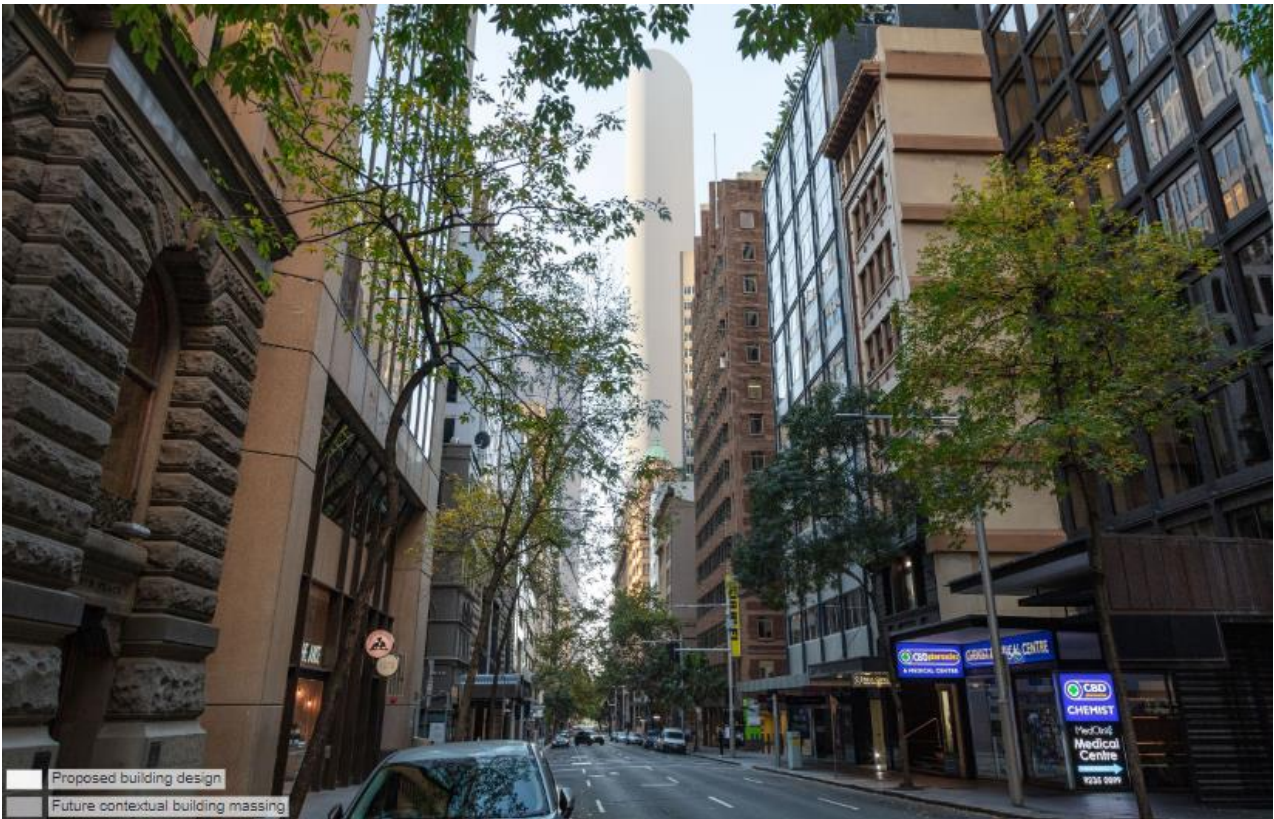
Figure 20 – View north along Pitt Street from Martin Place toward the subject site showing indicative massing of the proposed building in context. Source: Virtual Ideas, March 2024
